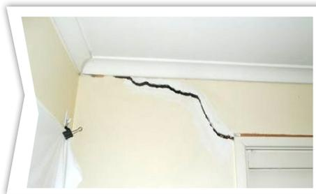
For prevention, there are a number of strategies that can be considered during the building process. For example, in seaside areas where there is sandy soil and a sloping site, it is smarter to build with suspended timber floors rather than on a concrete slab.
