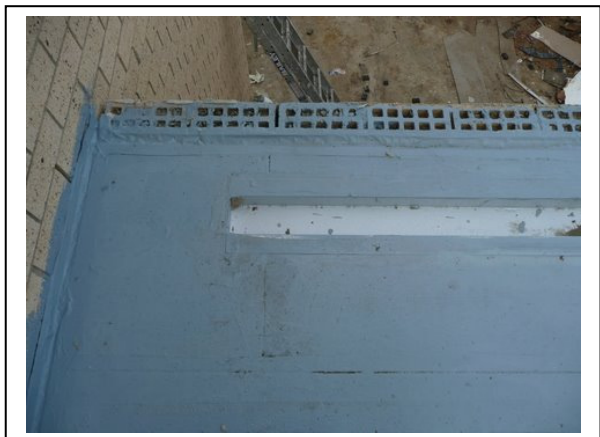
Waterproofing membrane to balcony over Garage
