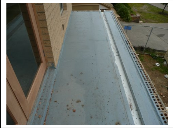
Waterproofing membrane to balcony off Bedroom 1
