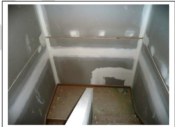
Expansion joint to plaster between storeys
