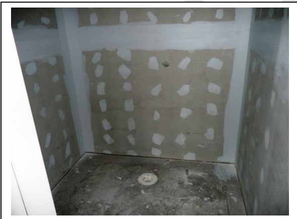
Waterblock sheeting to wet areas
